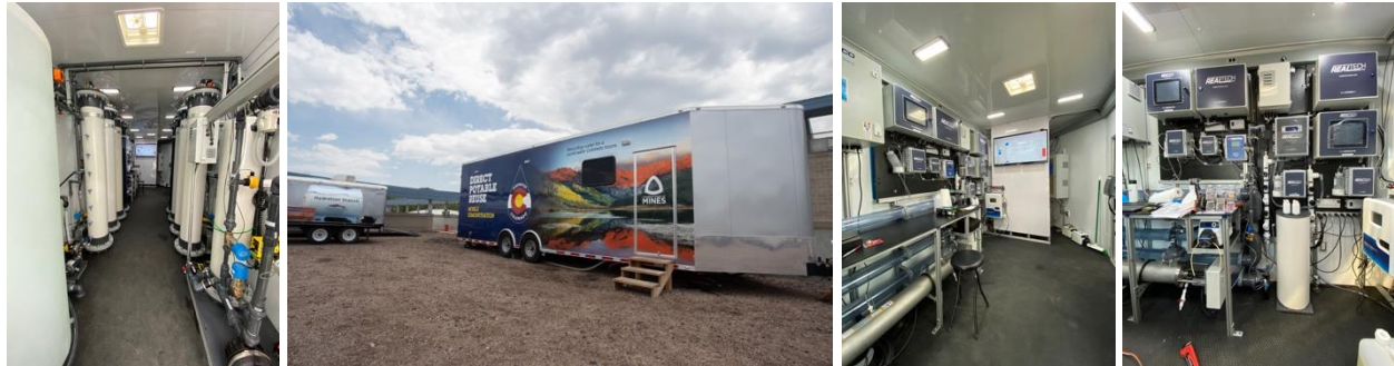
Figure 1: Scheme of the DPR pilot, including six unit processes: biologically active filtration (BAF), ozonation, ultra-filtration (UF), granulated activated carbon (GAC), UV treatment, and chlorination.
